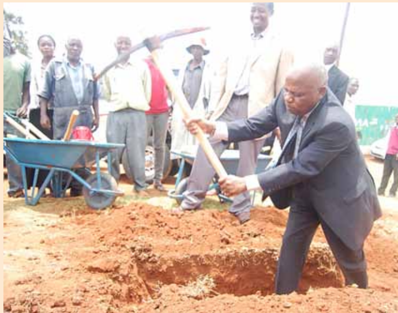
KNLS Board Chairman Mr. Silas Kobia breaks the ground for the construction of Kibera Community Library
